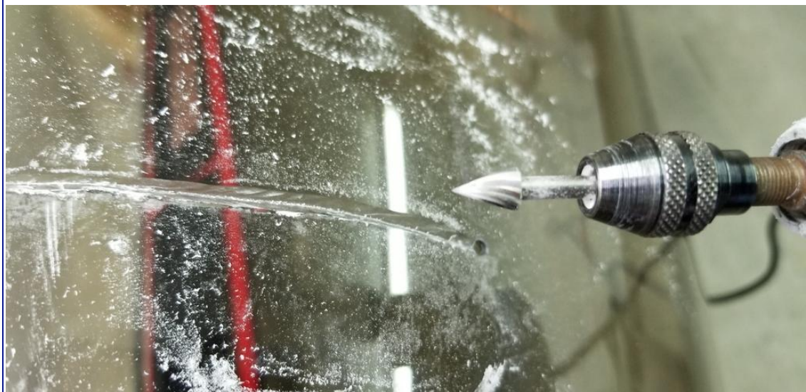
A Dremel #125 V-groove bit was used to begin the process of opening up the crack channel and relieving some of the built-in stress on the acrylic.
